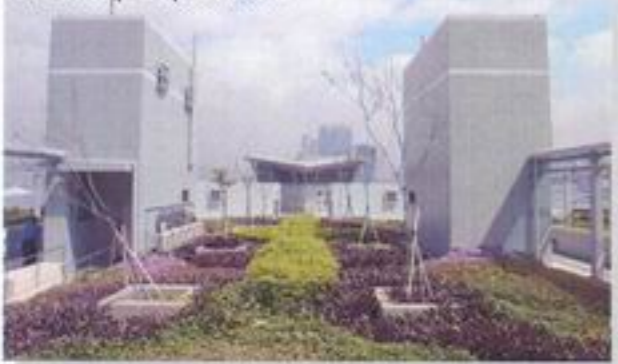
Roof top of pier no.2
