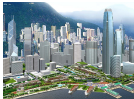
Figure 10 An integrated design of waterfront open space (Source: The New Central Harbourfront )
